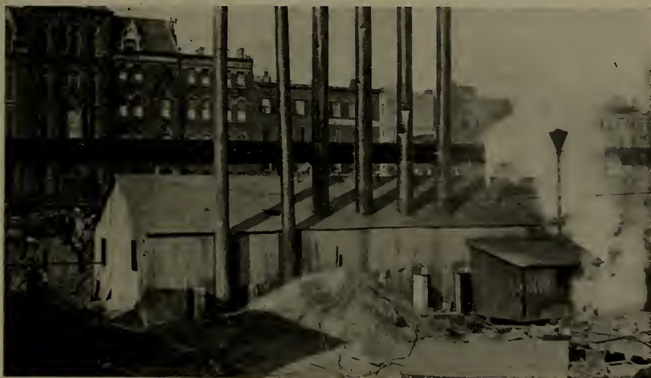
FIG. 1.—Temporary Power House, Pennsylvania Terminal.
